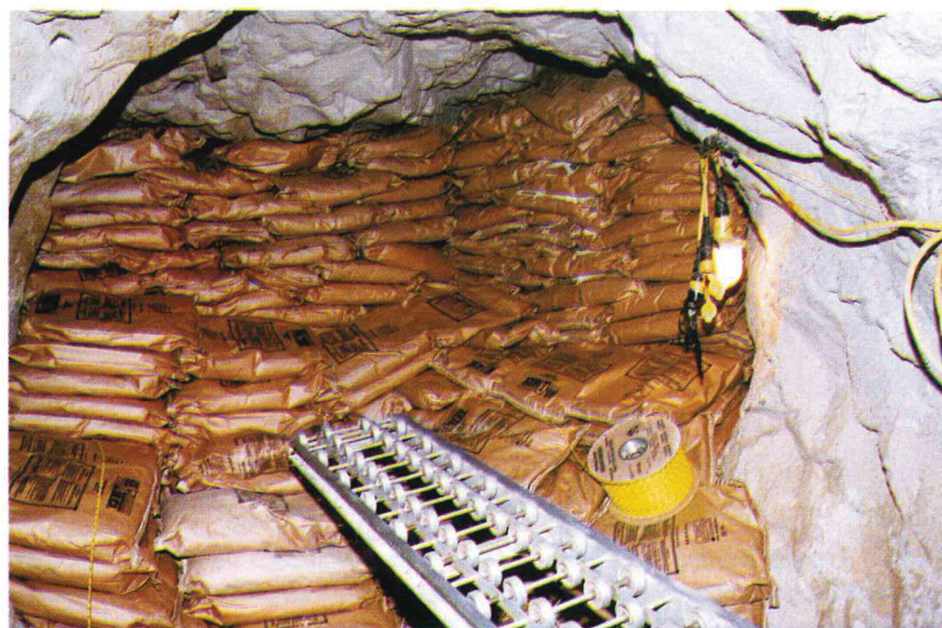
Bags of stemming—16,500, 40-lb bags of silica sand—were tightly packed in the ends of tunnels and adits in order to contain blast energy within the rock mass. Photo by John Freymuller.
