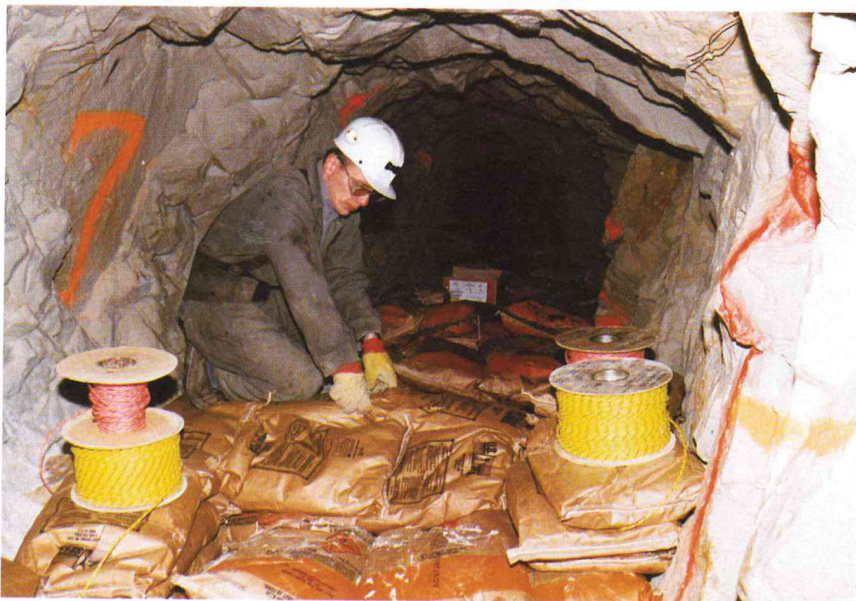
A blaster kneels on the end of an ANFO powder column, which formed a continuous explosive column in each tunnel. Powder factor was controlled by the height to which bags were stacked. Four lengths of reinforced detonating cord were used to provide a 4x-redundant initiation system in each tunnel. Cord and non-electric shock tubes were protected by carefully placed bags. Photo by John Freymuller.
